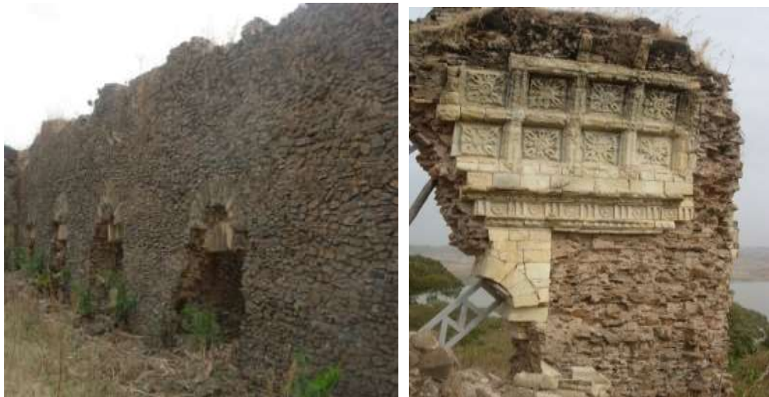
Part of the Remaining Building of Gorgora Nova.
